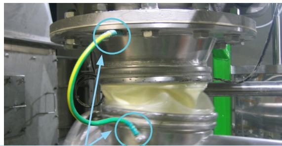
**IMPORTANT:** the metal connections on earthing/grounding cables need to be kept clean and tightly secured to ensure effectiveness.
